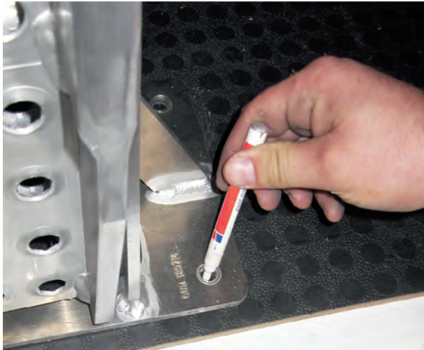
Figure 3: Marking the Fastening Holes
