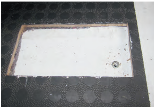
Figure 6: Floor Covering with Cut-Out for Installation Plate.
