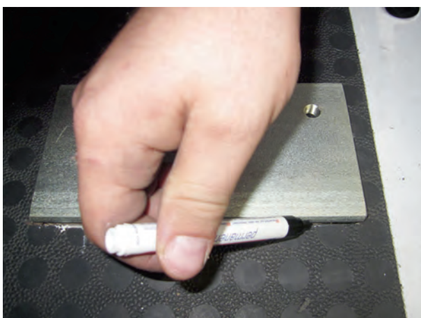
Figure 5: Marking the Installation Plates
